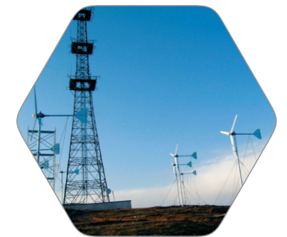
Telecom Base Station
